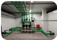
6. Pressure Pump Room with speed shifters
