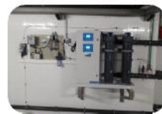
4. Saltwater chlorinator and control station
